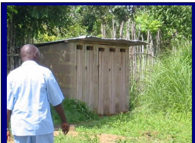
Adjacent Boys' and Girls' toilets (Gbalamuya Primary School)
