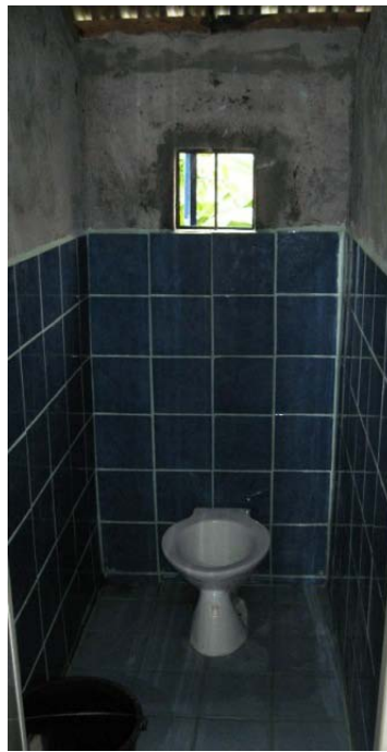
Toilets in Malilipot DCC
