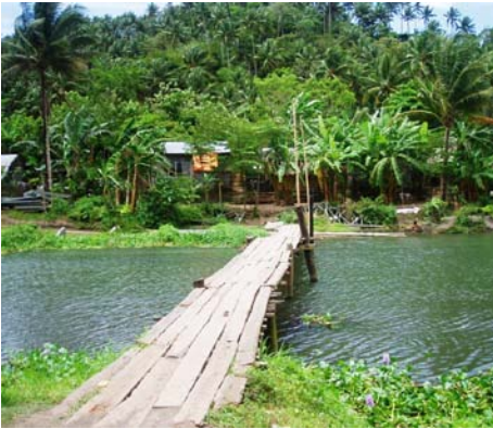
Make-shift bridge to Minto DCC
